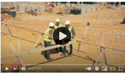
Construction Updates Jan 2021 LaVerde New Capital
